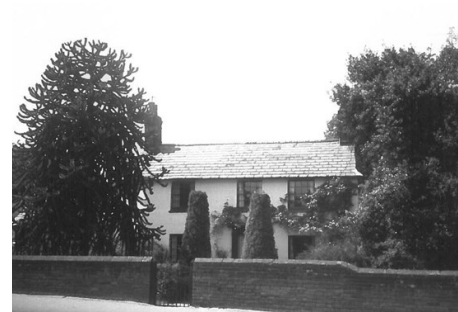
Figure 16 383 Old Road in 1985 (Essex County Council)
